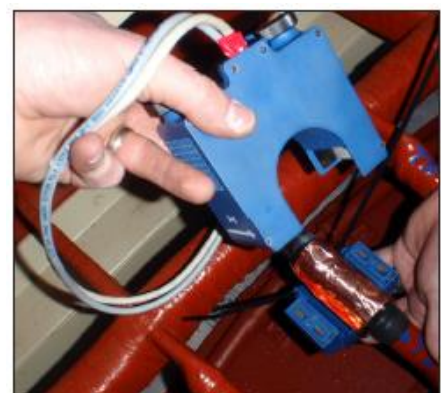
Figure 7: Assembling a 50-100H Current Transducer Head on a winding link of an Electrical Generator Stator. Reprinted by permission from the USBR.
