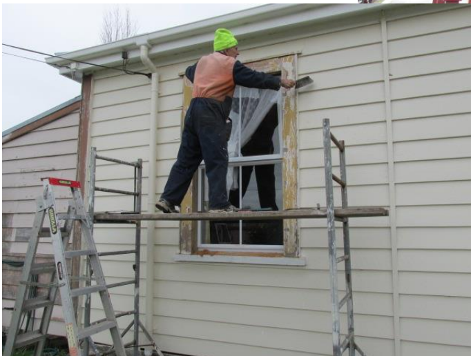
Barry Scott installing a new window
