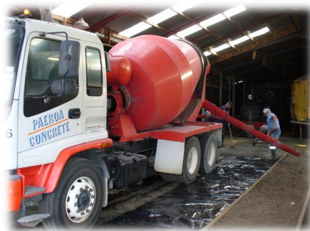
Pouring the Concrete
