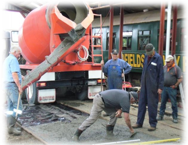
John laying concrete (with the assistance of some 'observers')
