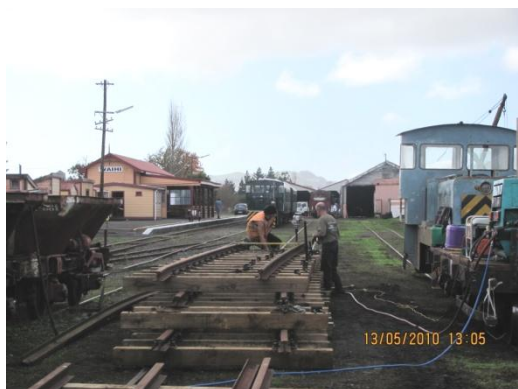
Building the reverse curve sets
