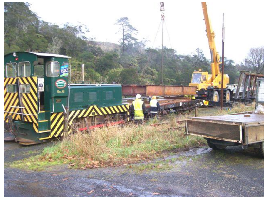
Removal of steel girder from No.8 Bridge
