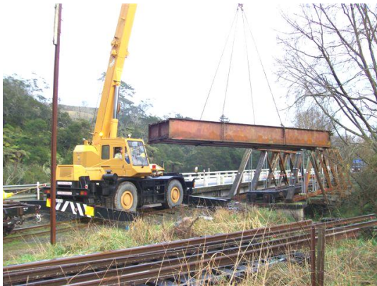
Removal of steel girder from No.8 Bridge
