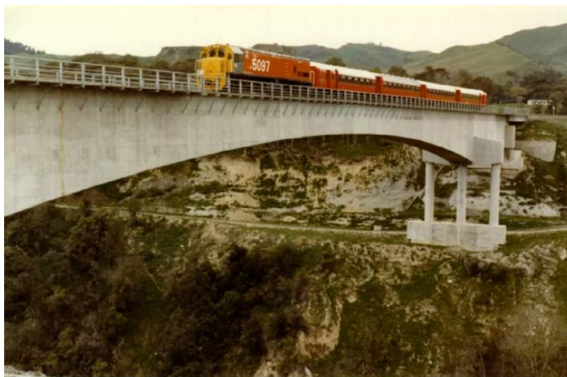
Kawhatau Viaduct – the 6 th the highest railway bridge
