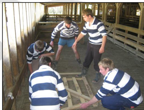
Palmerston North Boys High School Building a Gate - Overall Winners!
