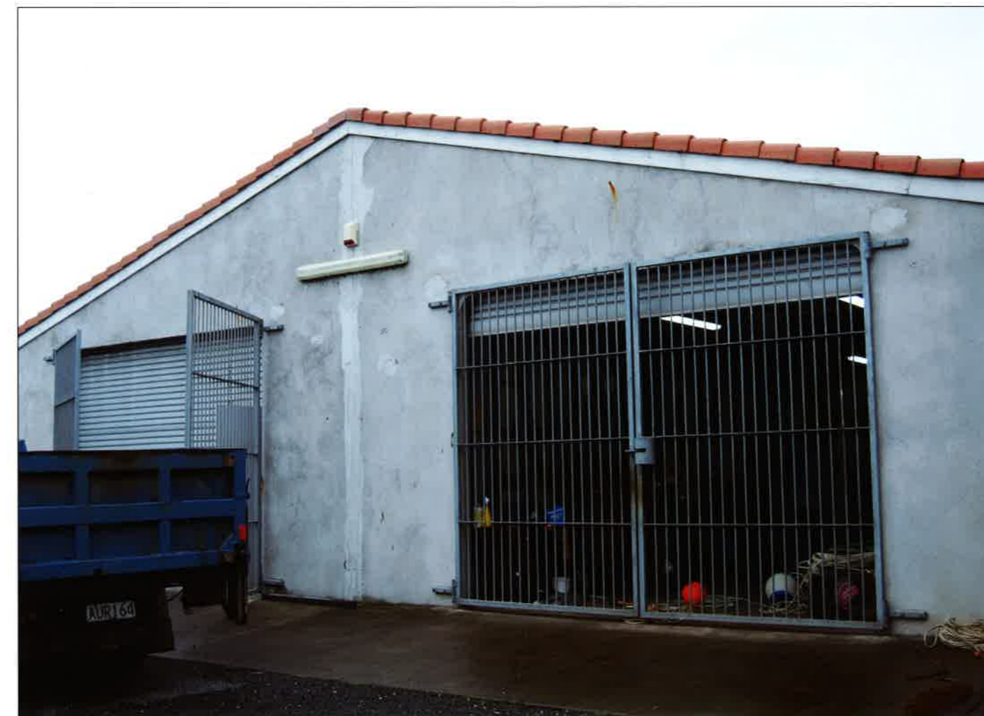
The team have a separate building for storing their cray pots and other gear, along with a workshop for maintenance.
